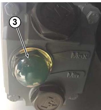
Fig. 19: Checking the oil level
